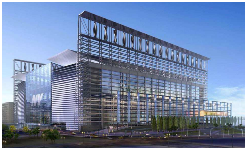
Rys. 11. Budynek New York Sports and Convention Centre [9]
